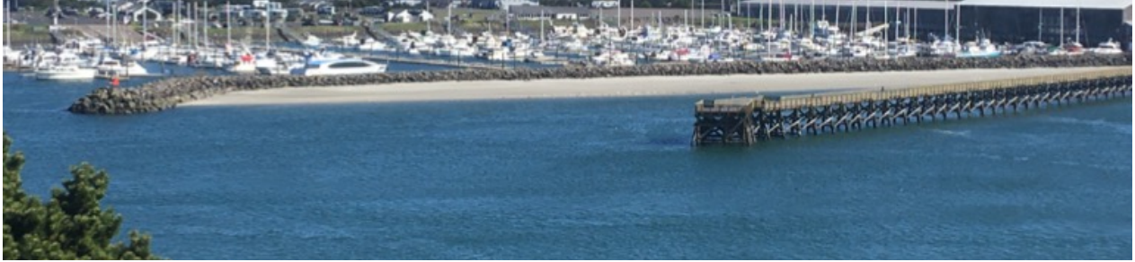
Sand collecting against breakwater at South Beach Marina
