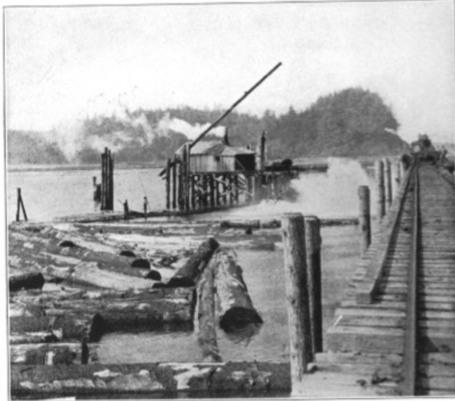
THIS VIEW SHOWS THE LOGS AT THE DUMP FROM THE OUTER END WHERE THEY ARE THROWN INTO YAQUINA BAY AND ALSO THE UNLOADING SHED AND ELEVATED "PILE" WHICH CARRIES THE LINE ABOVE THE LOGS
