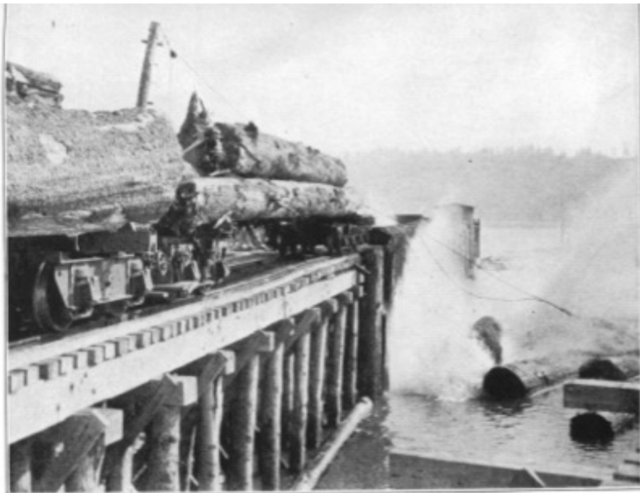
THE ABOVE VIEW SHOWS THE FINAL DUMPING SPOT AT OR NEAR THE END OF THE GREAT DOCK WHERE THE LOGS ARE UNLOADED THAT COME FROM HEAD-QUARTERS CAMP 1
