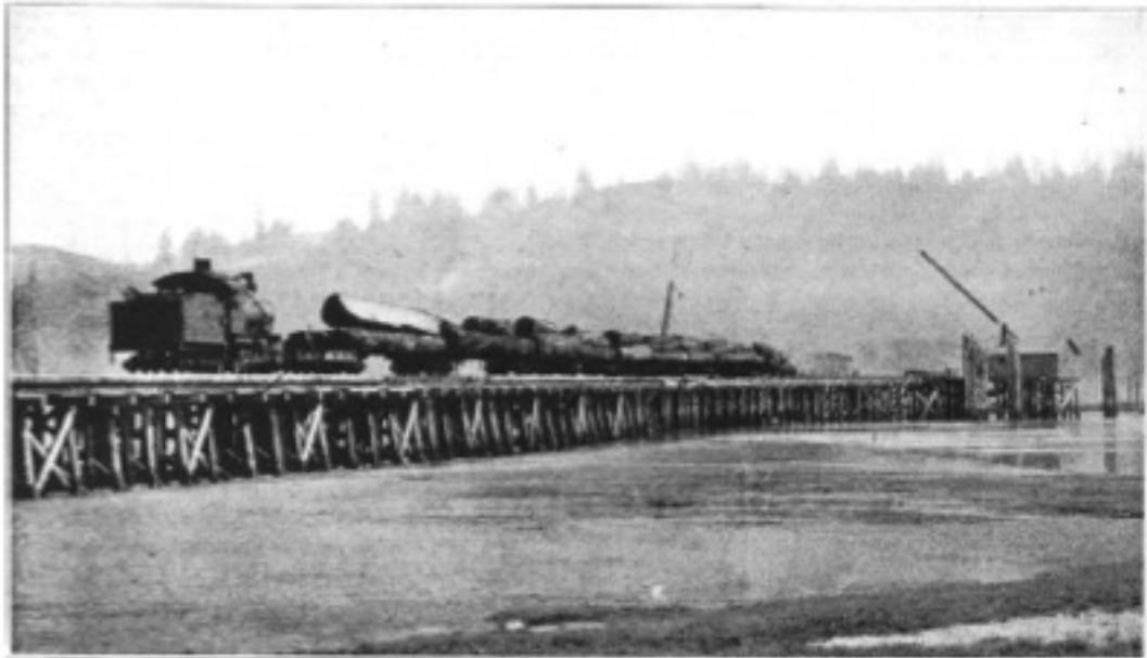
TEN CARS OF LONG-LENGTH SITKA SPRUCE AND OLD GROWTH YELLOW DOUGLAS FIR LOGS AT THE DUMPING WATERS AT SOUTHBEACH, OREGON, LOOKING OUTWARD FROM THE SHORE WITH LOCOMOTIVE PUSHING THEM INTO PROPER PLACE FOR DUMPING
