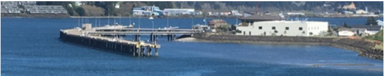
NOAA facility and dock at South Beach
