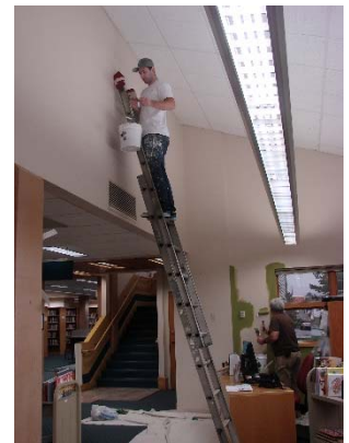
Newport Library Renovation
