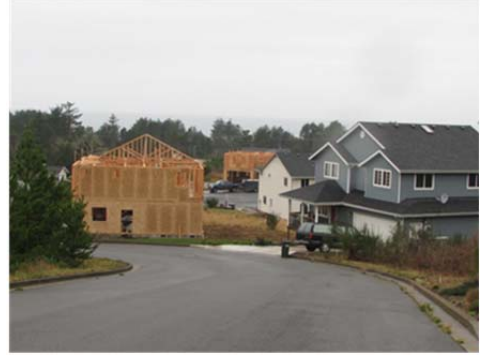
N.E. 71st and Avery Housing Construction
