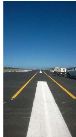
Airport Runway Reconstruction
