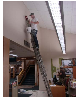
Newport Library Renovation
