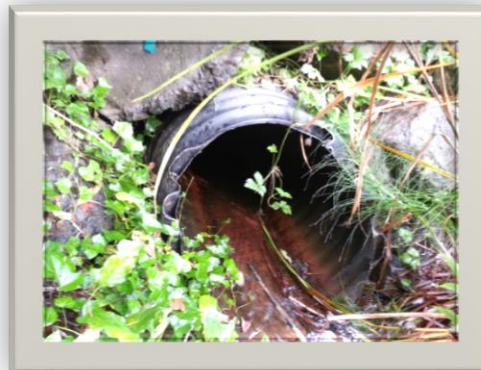
Figure 3.41 – Image of culvert Q1-C
