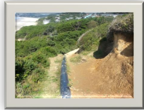
Figure 3.15 – Image of Outfall S1
