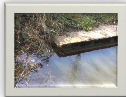
Figure 3.27 – Image of Outfall AG2
