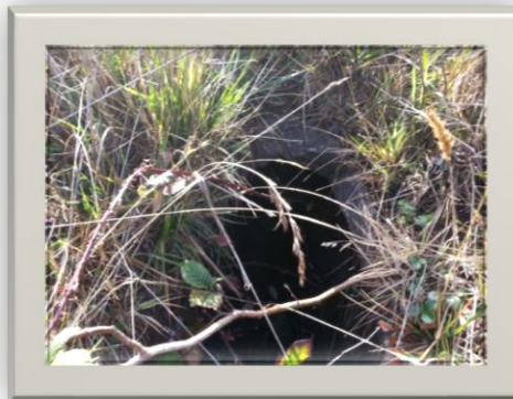
Figure 3.56 – Image of Culvert AP1-C
