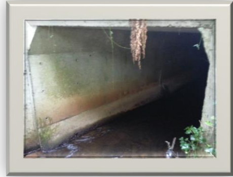
Figure 3.32 – Image of Outfall AN1
