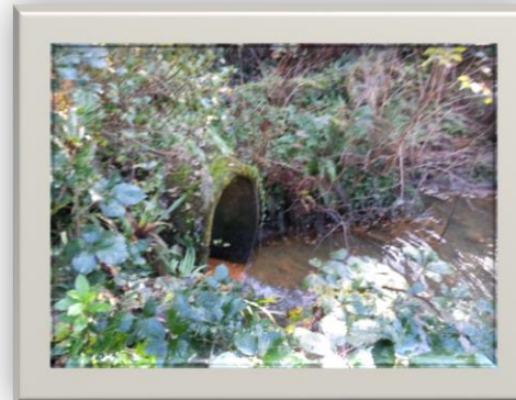
Figure 3.44 – Image of Culvert U1-C
