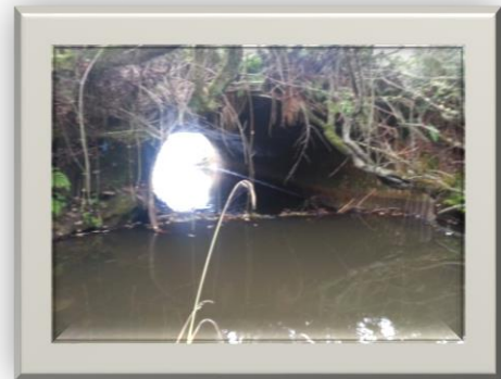
Figure 3.11 – Image of Outfall N1
