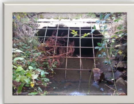
Figure 3.50 – Image of Culvert AG5-C
