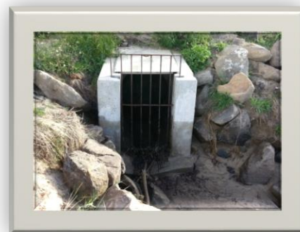
Figure 3.26 – Image of Outfall AF1
