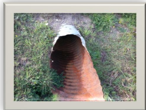
Figure 3.52 – Image of Culvert AL1-C1
