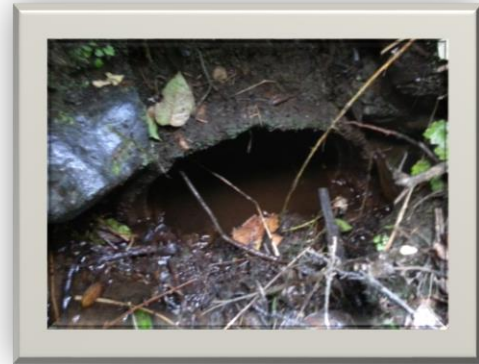
Figure 3.58 – Image of Culvert AP4-C
