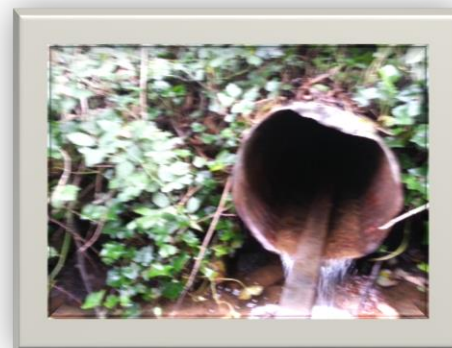
Figure 3.14 – Image of Outfall Q1
