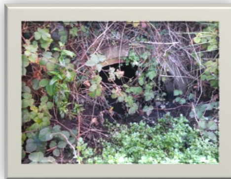
Figure 3.48 – Image of Culvert AG3-C
