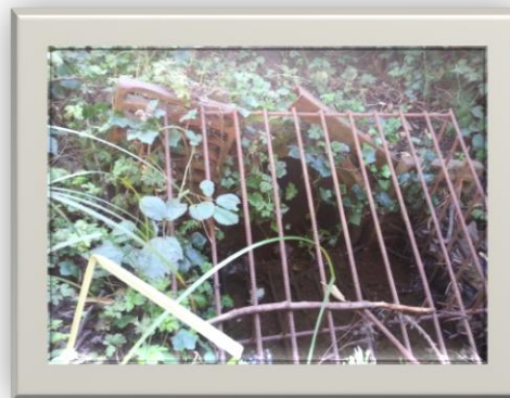
Figure 3.43 – Image of culvert T2-C
