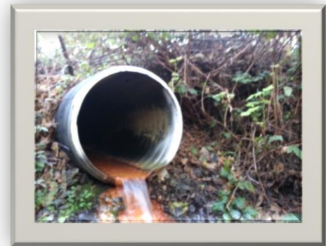
Figure 3.4 – Image of Outfall B1
