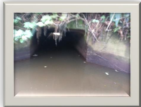
Figure 3.33 – Image of Outfall AO1
