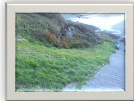
Figure 3.18 – Image of Outfall V1
