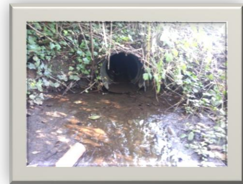
Figure 3.47 – Image of Culvert U4-C
