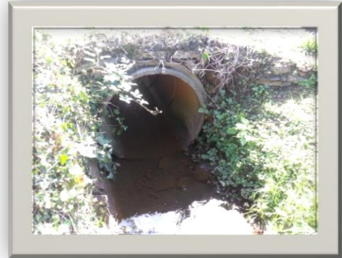
Figure 3.45 – Image of Culvert U2-C
