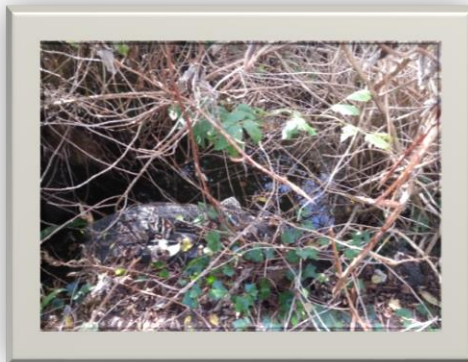
Figure 3.49 – Image of Culvert AG4-C
