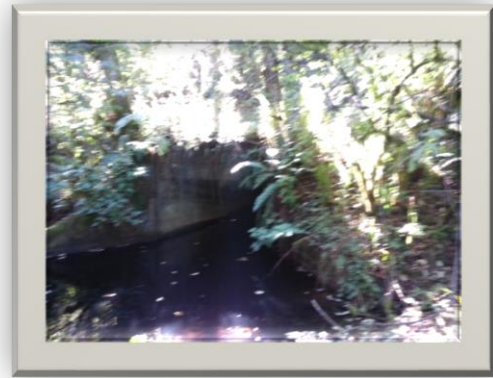
Figure 3.38 – Image of culvert M1-C
