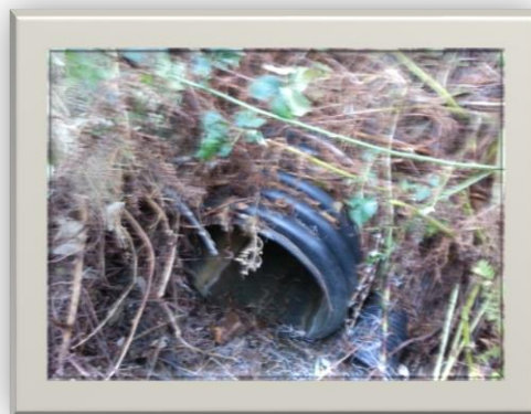
Figure 3.36 – Image of culvert G1-C
