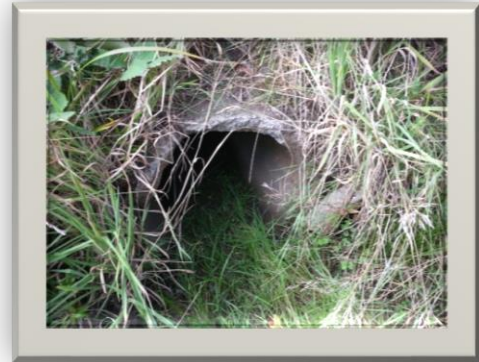
Figure 3.51 – Image of Culvert AG6-C
