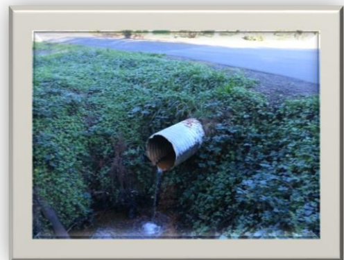
Figure 3.39 – Image of culvert N1-C
