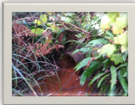
Figure 3.57 – Image of Culvert AP2-C
