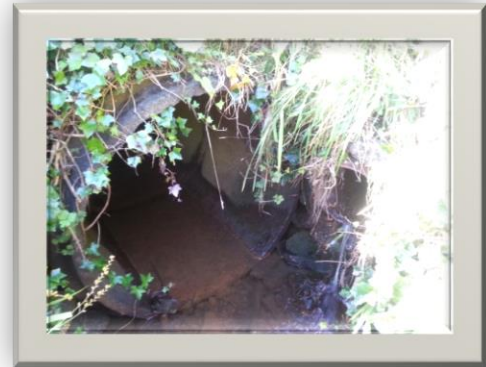
Figure 3.46 – Image of Culvert U3-C
