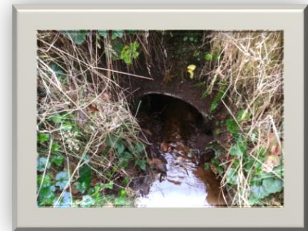
Figure 3.29 – Image of Outfall AJ1
