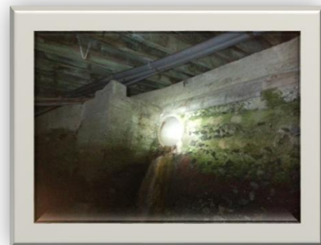
Figure 3.22 – Image of Outfall AA1
